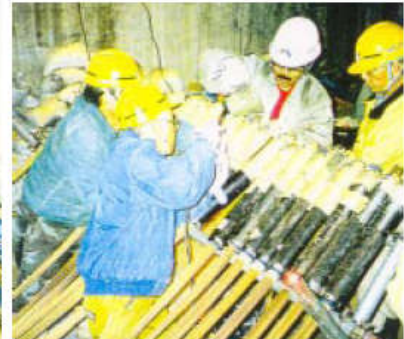
Injection of mortar into the tendon mounted anchorages.
