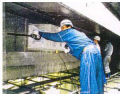
Installation and jacking of external steel cables.
