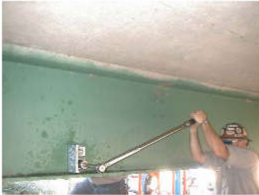
(a) Installation of anchorage assembly
