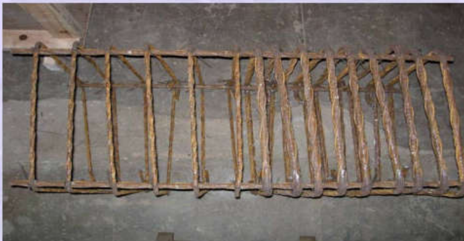
(a) Fabrication of end zone reinforcement
