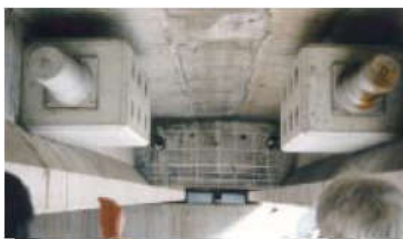
End view of anchor blocks with external cables and anchorages.
