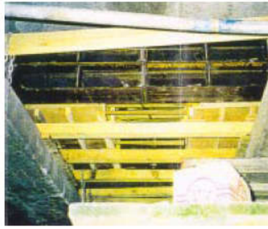
Placement of temporary reaction devices between girders.
