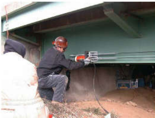
(c) Application of P-T force in West-end span
