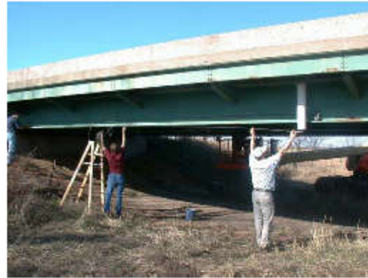
(b) Placement of CFRP rod
