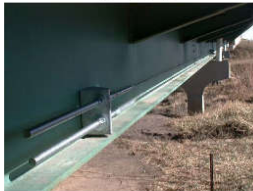
CFRP Rods on span
