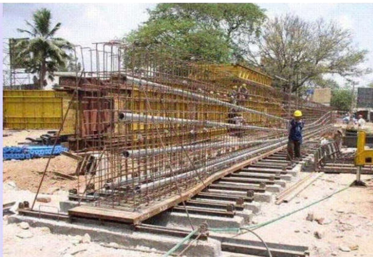
(a) Fabrication of reinforcement
