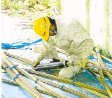
Preparing the anchorage (bond-type)
