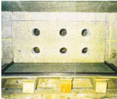
Drilling of holes into girders for the introduction of aramid tendons.
